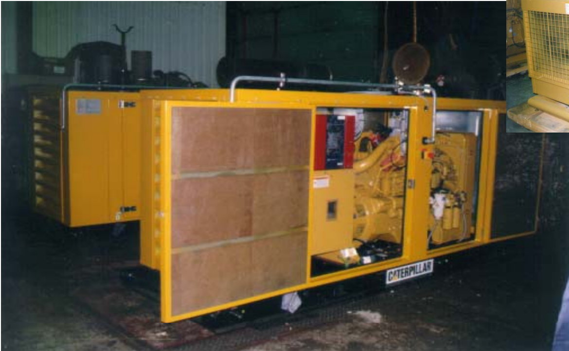
(Above) The 3304 DIT generator set with EMCP and secondary shutdown system
