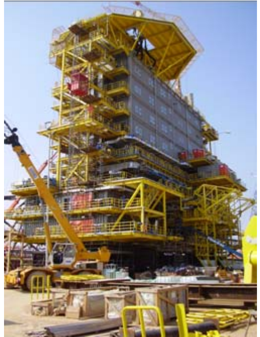
Working on the Halfdan BC platform
