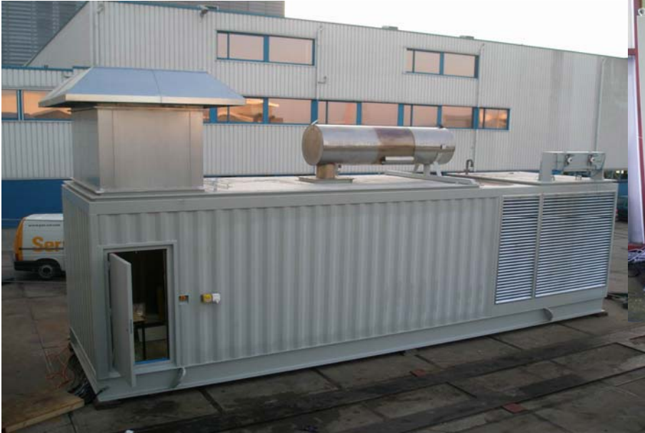
(Above) Complete unit during FAT at workshop in The Netherlands.
