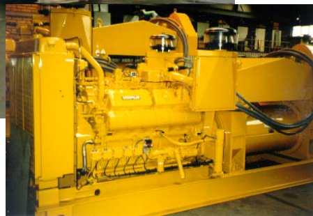
(Below) 3412 DITT Caterpillar packaged with IP55 air to air cooled Leroy Somer generator
