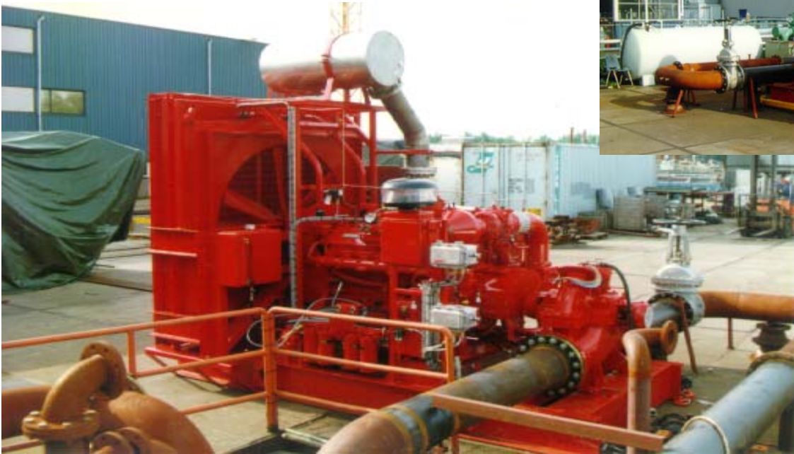
(Above) Presurized control panel and extra large radiator for additional cooling in high temperature environment
