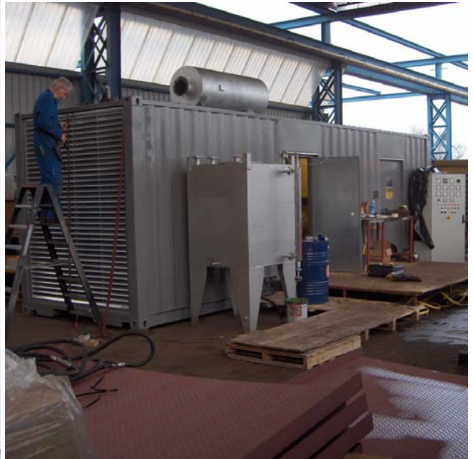
(Above) Preparation for FAT testing in workshop.
