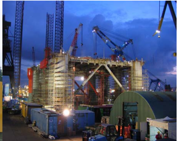
(Above) Blackford Dolphin drill rig under construction at shipyard
